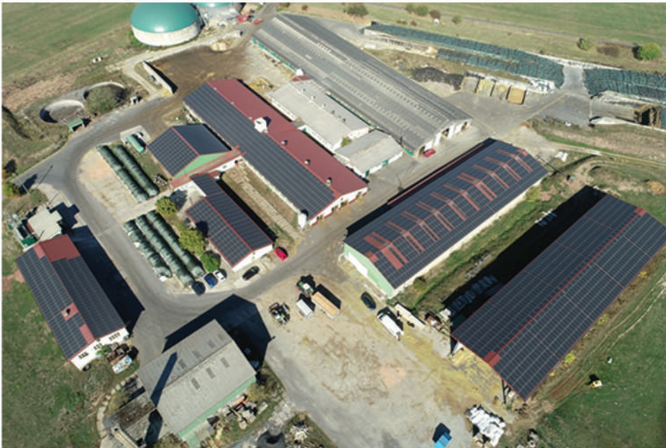
Crock MVA 750kWp, Germany
