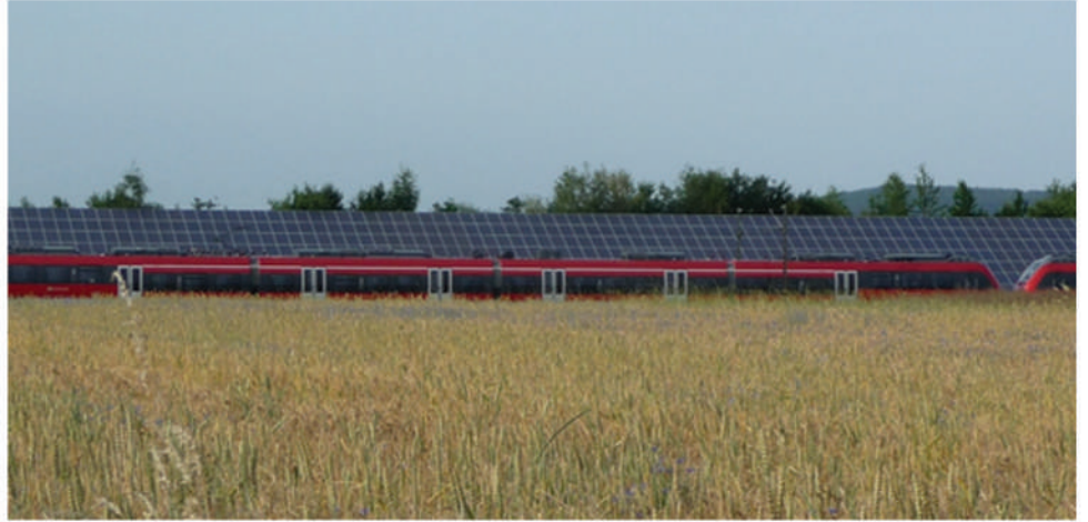
Noise protection wall Neumarkt idOPF. 1227kWp, Germany
